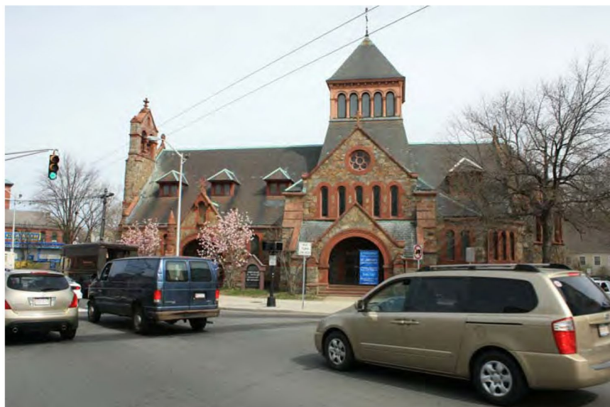
2 Church Side Facing Corner Of Mass. Ave and Beech St.
