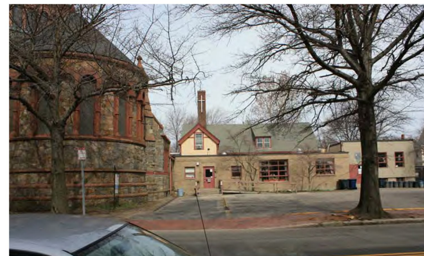
6 Church Side and Parish House Fronting on Beech St.
