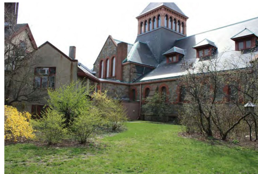
4 Church Rear (North Side)
