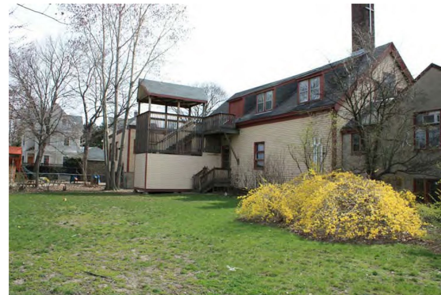
5 Parish House (North Side)
