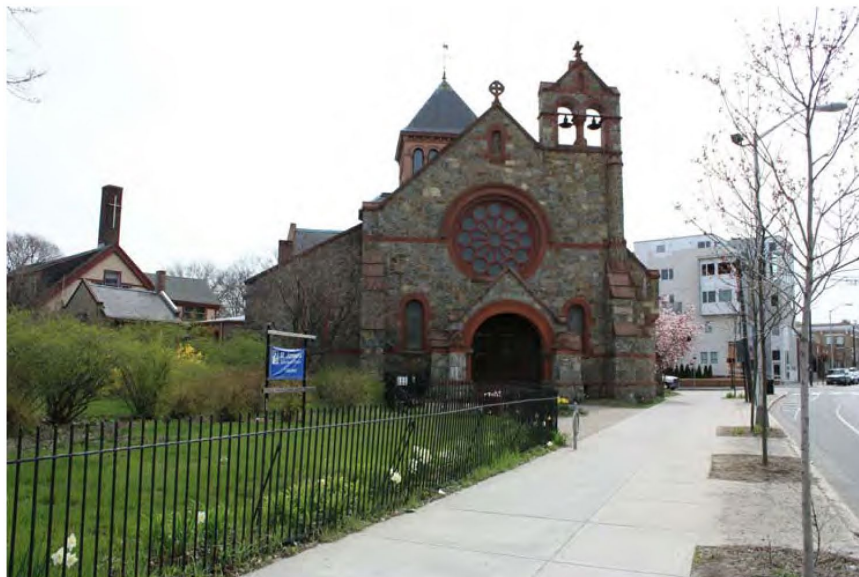
1 Church Front Facing Mass. Ave.
